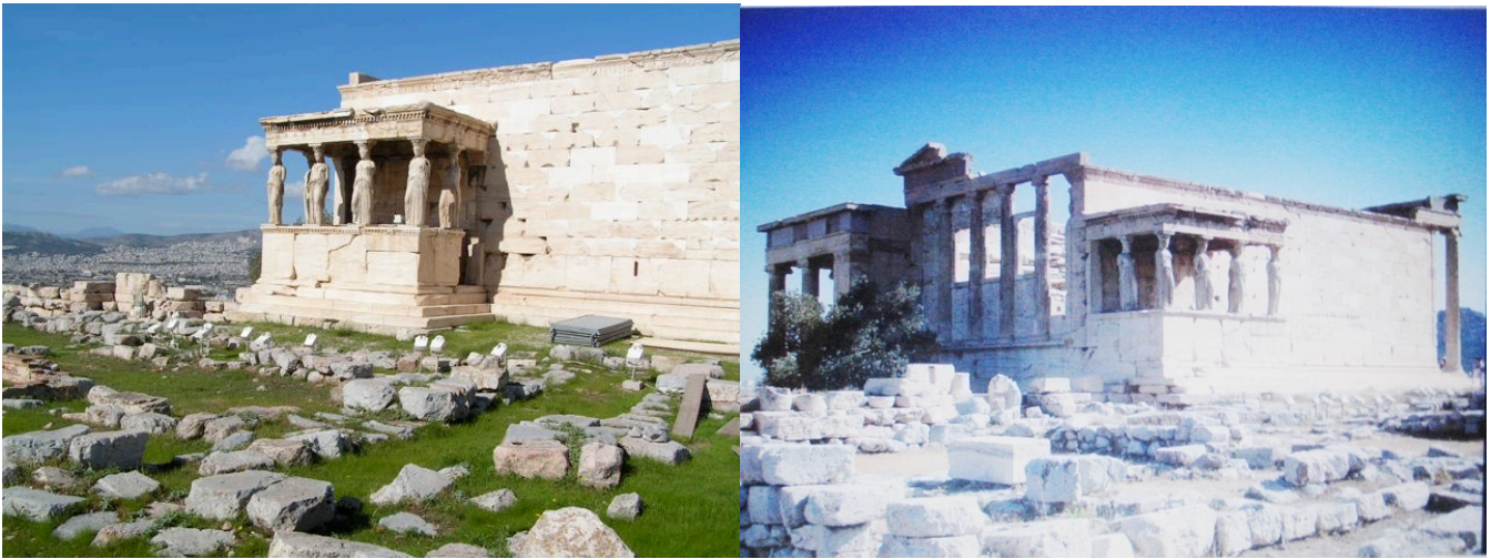
Figure 13 and 14. The Erechtheion (a Temple to both Athena and Poseidon) built between 421-406 BCE in Pentelic marble transported from Mt. Pentelicus, a distance of approximately 16km.
