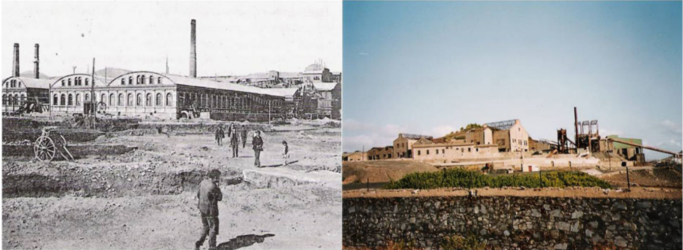
Figure 10. The ore flotation plant of the Greek company at the beginning of 20th Century. With a 3350 m 2 surface area it was then one of the biggest in the world. Unfortunately, only a small part of it was saved. (Image from the book "Historical and technological equipment in Greece")
